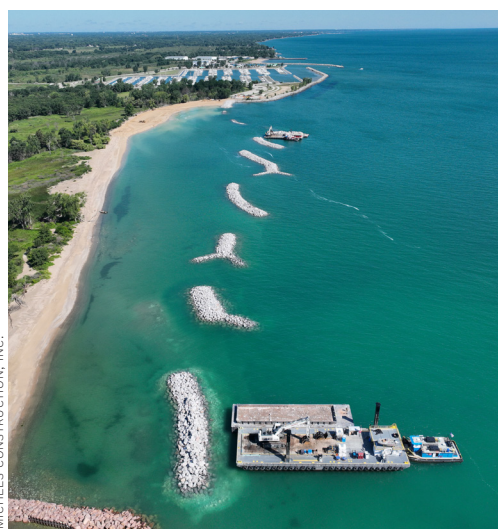
Beach and Breakwater Overview.
