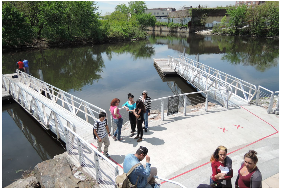
The WEDG Certified Starlight Park in the Bronx, New York provides a floating dock on either side of a weir, allowing boaters to navigate over or around the barrier at high and low tide. Photo: Jim Henderson
